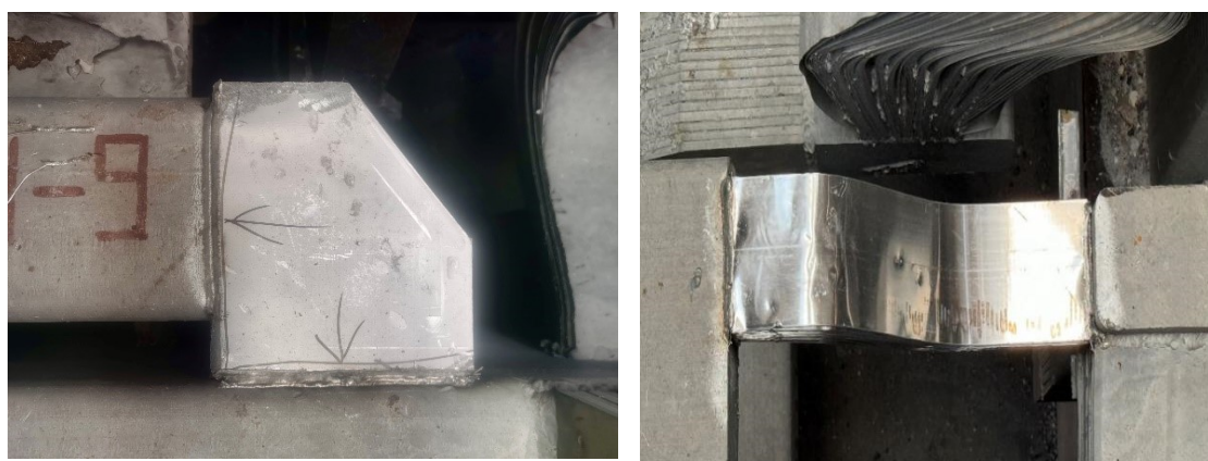
Figure 10. Welding quality of 420 kA optical-magnetic welding machine during construction.
